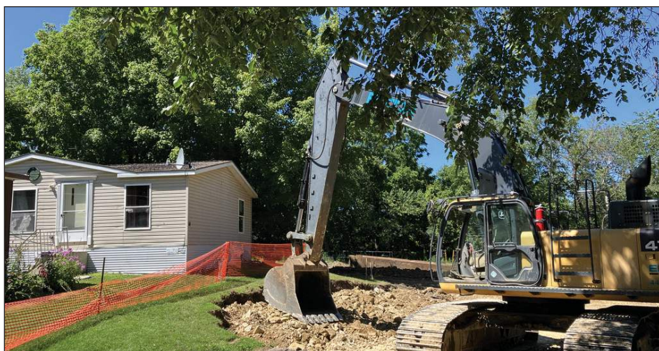
Zumbro Ridge installed several catch basins to redirect stormwater from their roads, one of several infrastructure improvement projects completed in recent years. Before the catch basins, the Co-op routinely spent thousands of dollars fixing road failure and erosion caused by stormwater.
