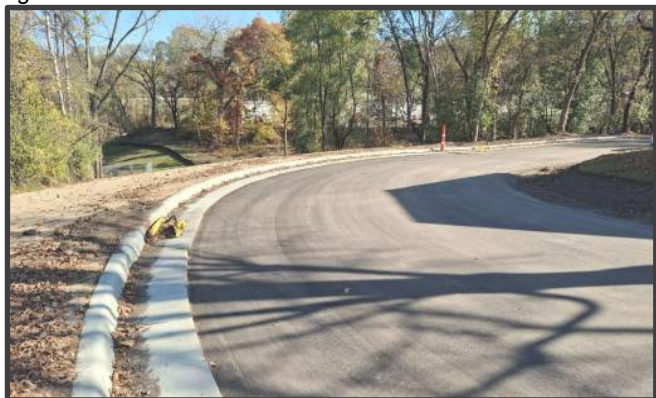
Culverts, curbs and catch basins at ZRE direct stormwater safely downslope beneath the future roadway, protecting against washouts and erosion.
