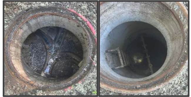
New sanitary sewer (left) and water system (right) manholes
