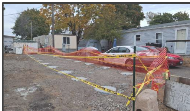
Below: Vacant lot prepped with concrete piers in preparation for a new single-section home in PPC.
