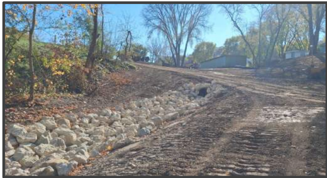
Culverts, curbs and catch basins at ZRE direct stormwater safely downslope beneath the future roadway, protecting against washouts and erosion.
