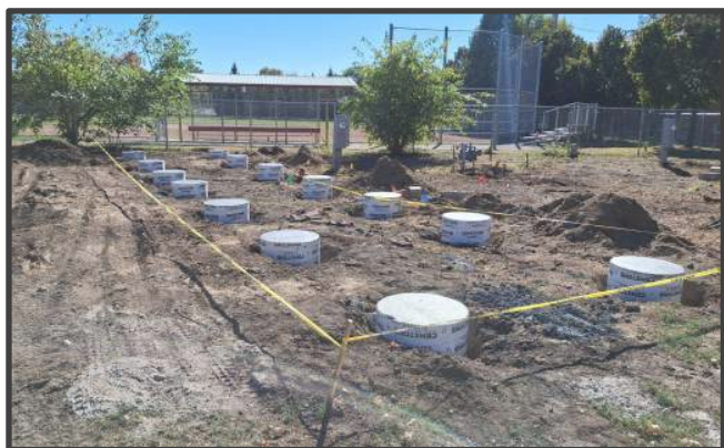
Concrete piers are set on vacant lots in preparation for a new single-section home for WTC.
